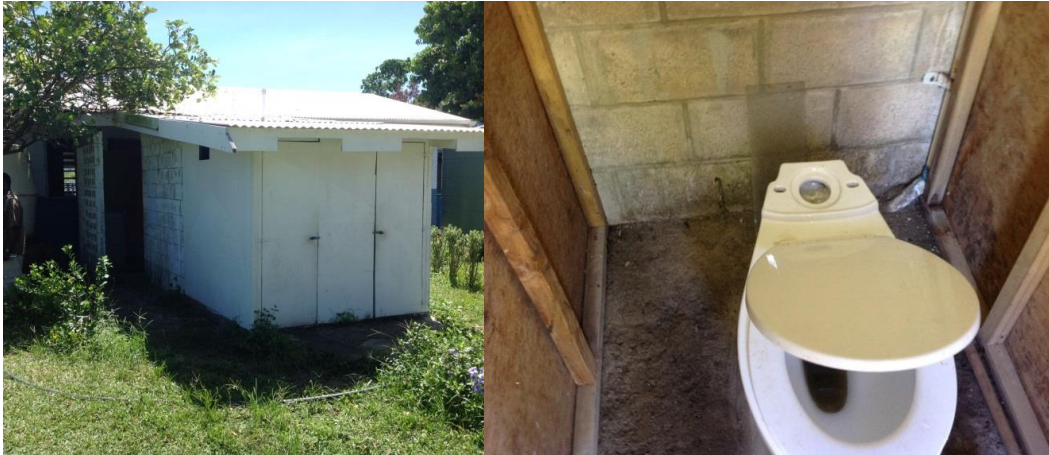
Before refurbishment – April 2017
