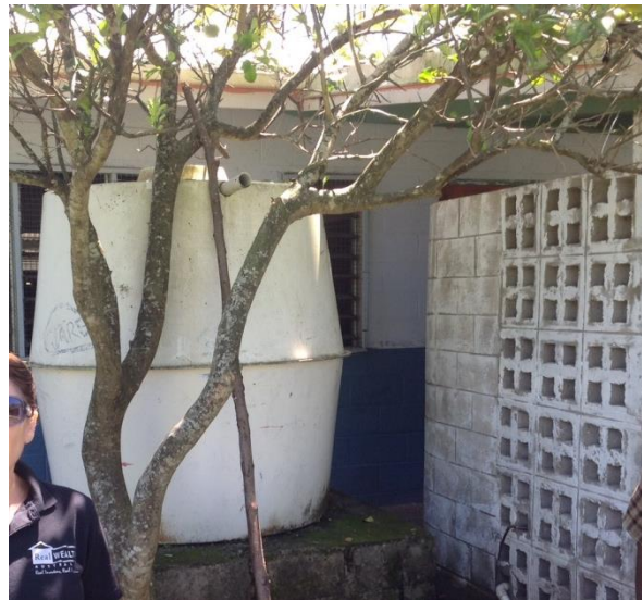
Water tank still needs to be raised higher on plinth to provide gravity feed alternative to flush toilets
